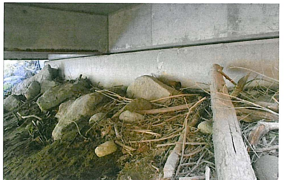
CK-2440 Left Abutment
