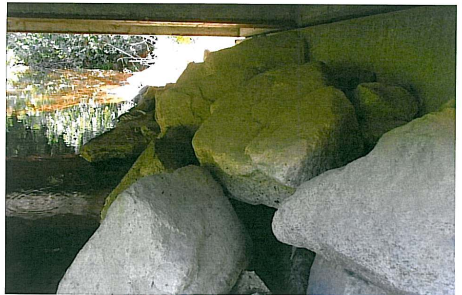
CK-2440 Right Abutment
